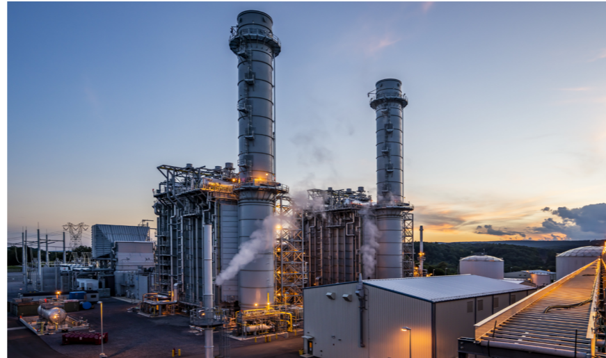
Fairview CCPP, USA
