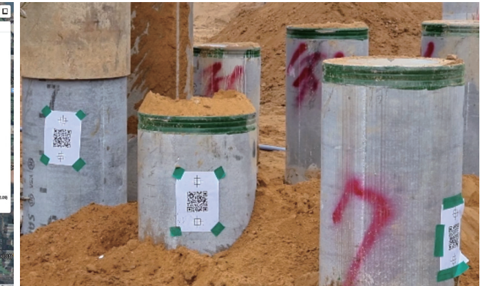
Camera-based Pile Rebound Value Check
