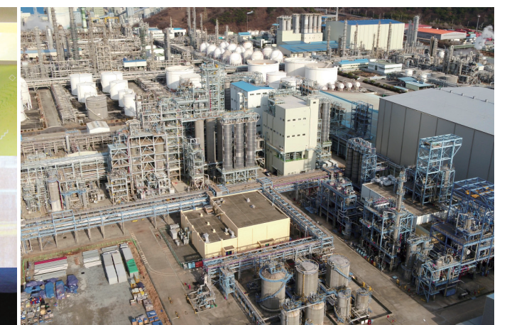
DL Chemical polyethylene plants in Yeosu, Jeollanam completed using the AWP
