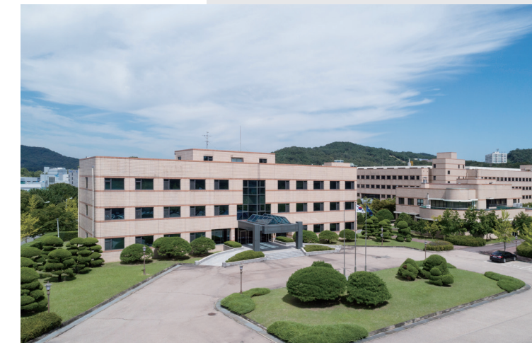
View of DL Chemical Daedeok R&amp;D Center
