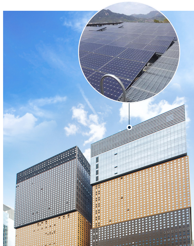
View of Solar Panels on the D-Tower
